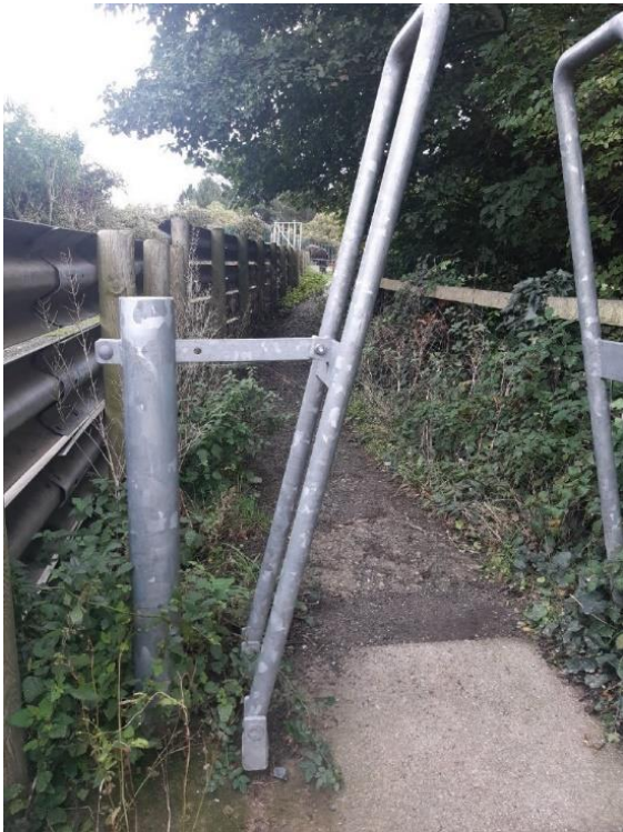
Figure 4-7: Adjustable A Frame Barrier Example – Point of Ayr
