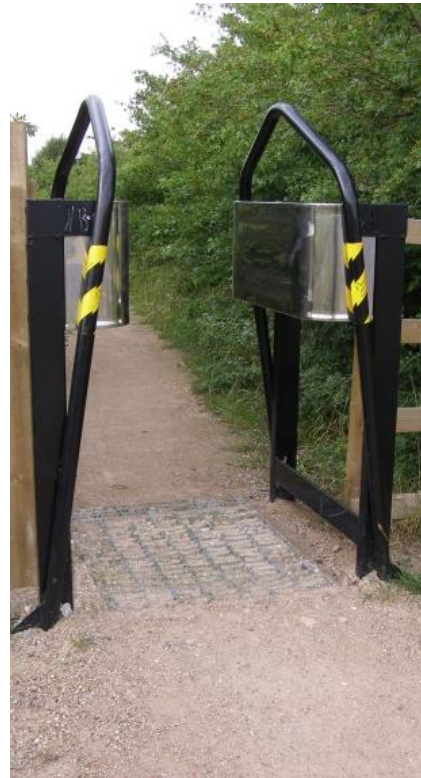
Figure 4-6: K Frame Barrier Example
